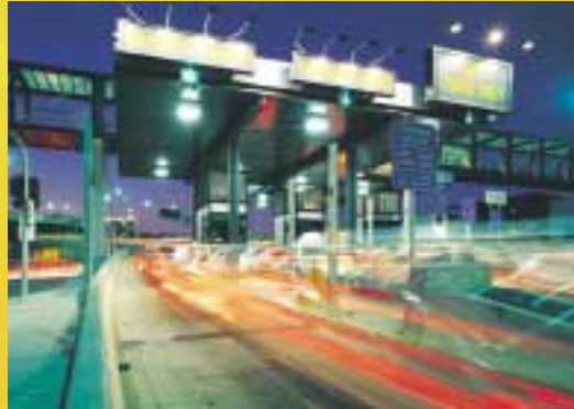
Eastern Distributor maintenance and operation Sydney, New South Wales
