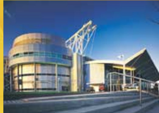
Mortlake rehabilitation New South Wales
