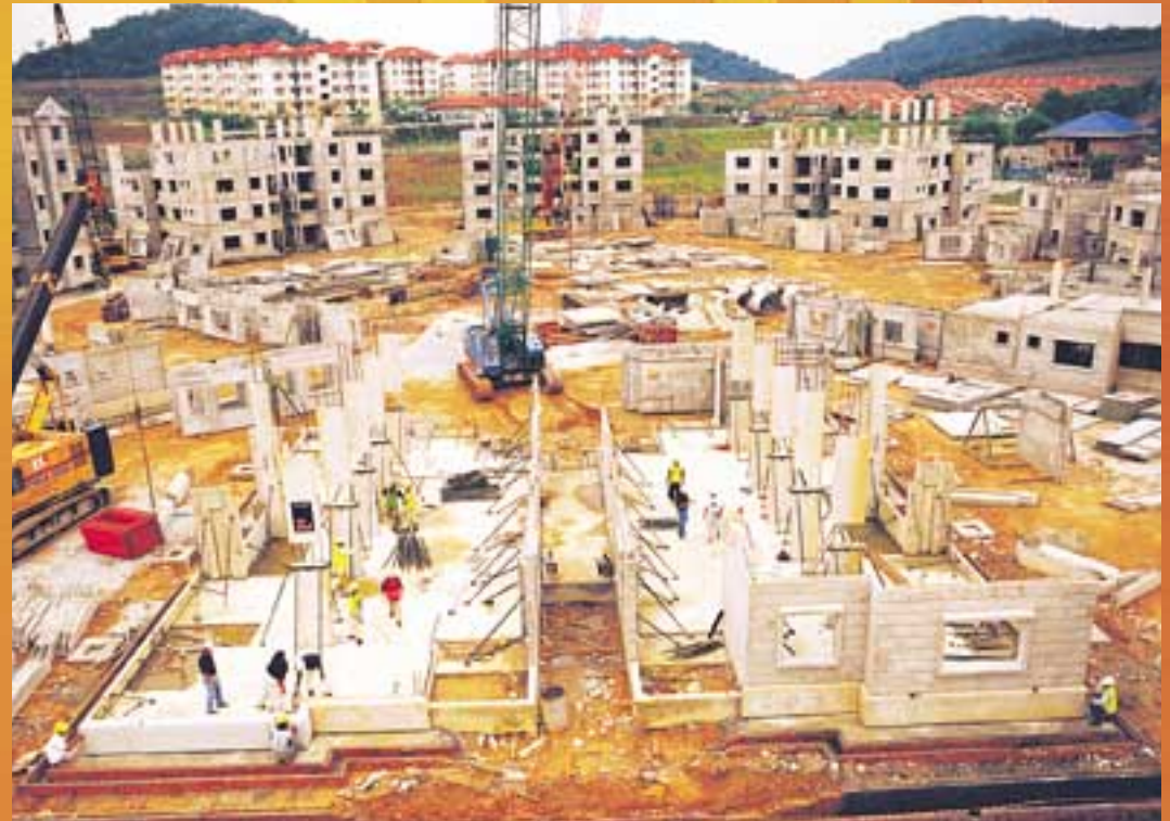
Teachers' Housing project Malaysia
