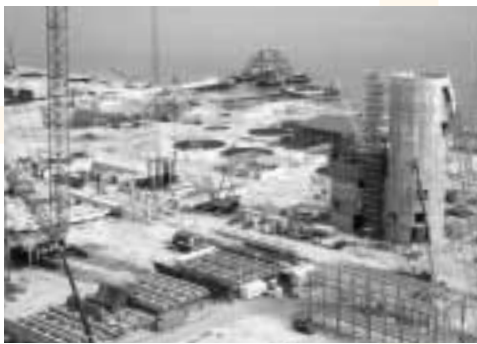
Far Left ABC Accommodation Building, Computer Rendering New South Wales, Leighton Contractors
