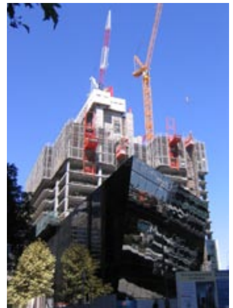
The glass curtain wall is now being put into place
