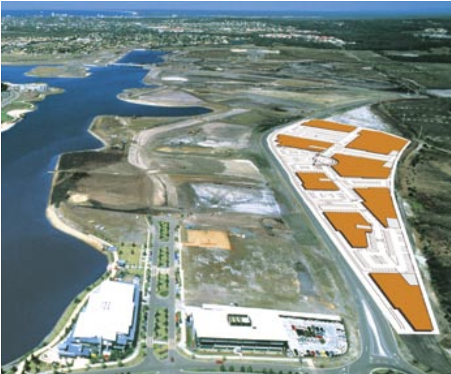
Aerial image of the Kawana project highlighting the eight individual building sites that comprise the development
