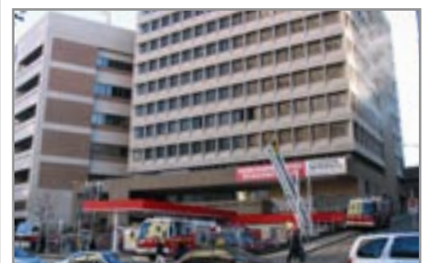
Activity surrounding 100 Pacific Highway by the NSWFB prior to demolition of the existing building
