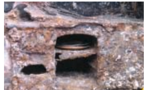
A cast-iron stove uncovered in the basement of one residential building still containing cooking utensils
