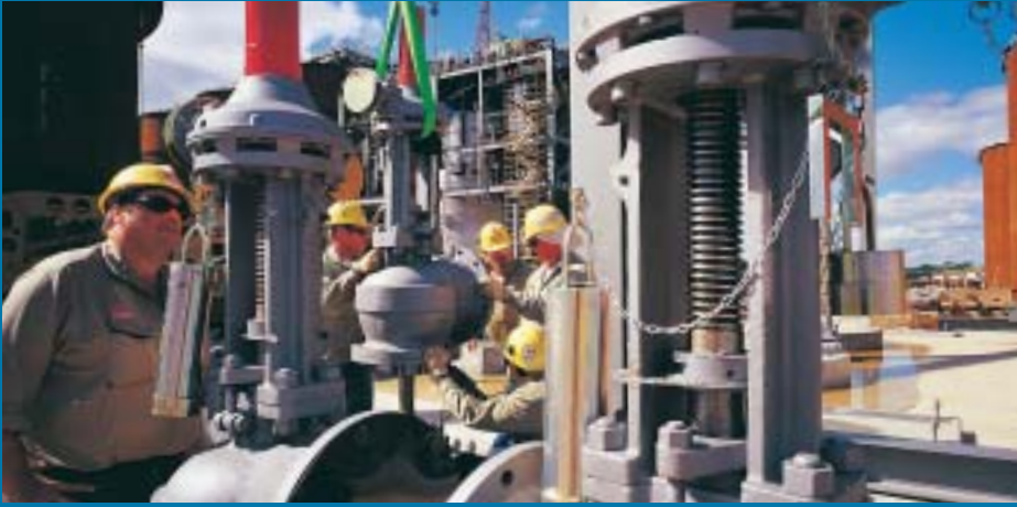
Comalco Alumina Refinery, Queensland John Holland
