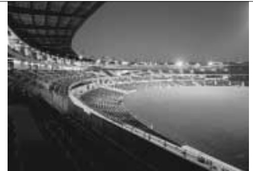
Above Subiaco Oval redevelopment Western Australia, John Holland
