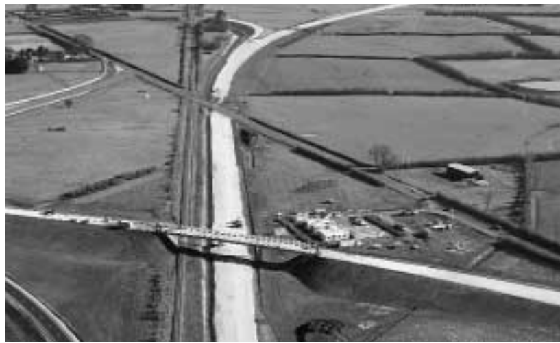
Bass Highway, Tasmania, Leighton Contractors
