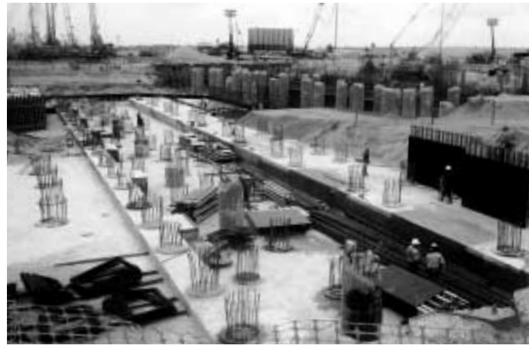
Manjung Power Station, Malaysia, Leighton Asia
